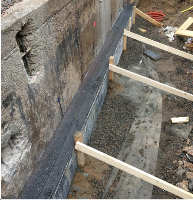
Figure 9. Newly cast vat with cast-in anode band (photo Öresundskraft).
