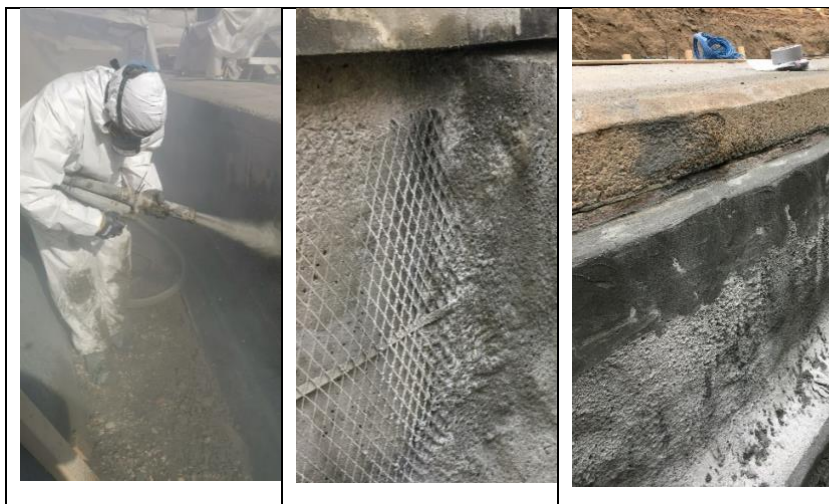
Figure 10. Spraying of anode mesh (photo Öresundskraft).
