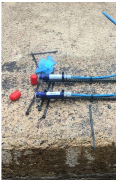
Figure 7. Reference electrodes of the manganese dioxide type that are attached to the reinforcement before concreting (photo Öresundskraft)
