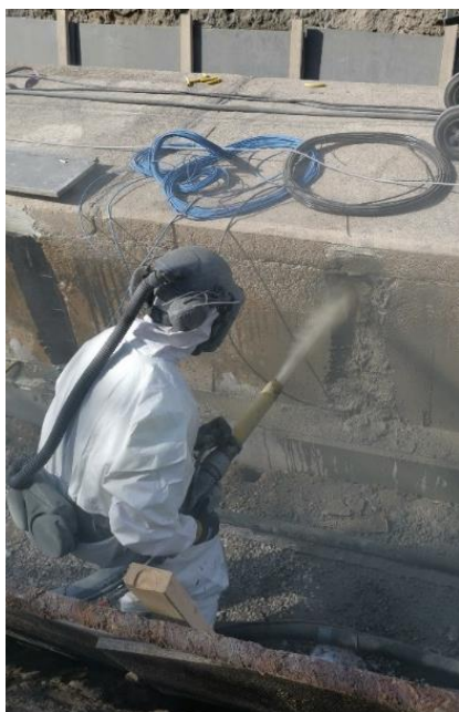
Figure 8. Repair of concrete damage and injection of mounted reference electrodes and cable connections. (photo Öresundskraft)
