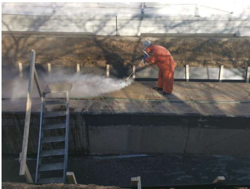
Figure 5. High-pressure washing of concrete culverts (photo Öresundskraft).
