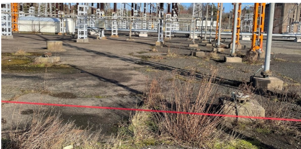
Figure 1 Ground at site with asphalt and foundations
