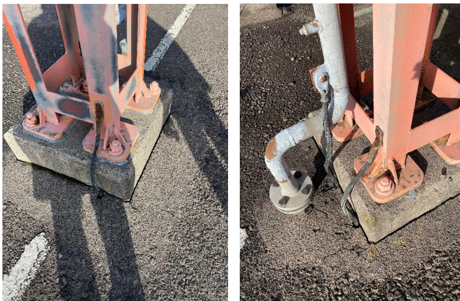
Figure 4 Connections to earthing grid
