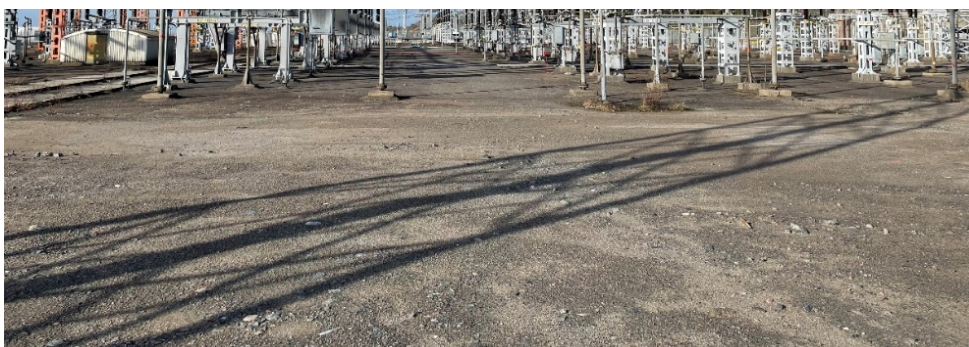
Figure 2 Ground at site with asphalt and foundations
