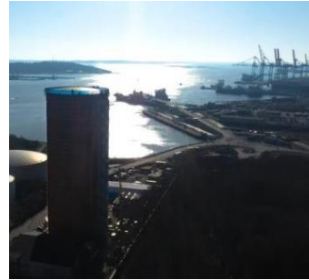
District heating with heat storage
