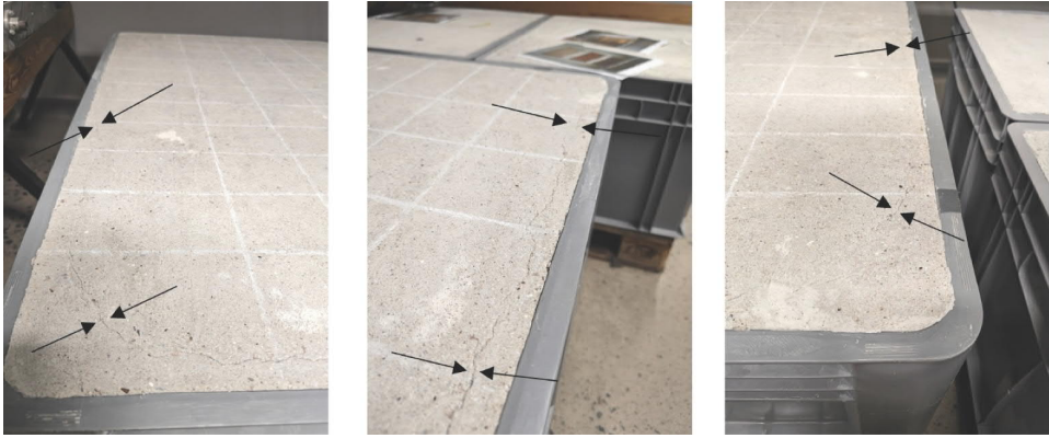
Figure 4. Surface cracks along the boundary of the specimen.
