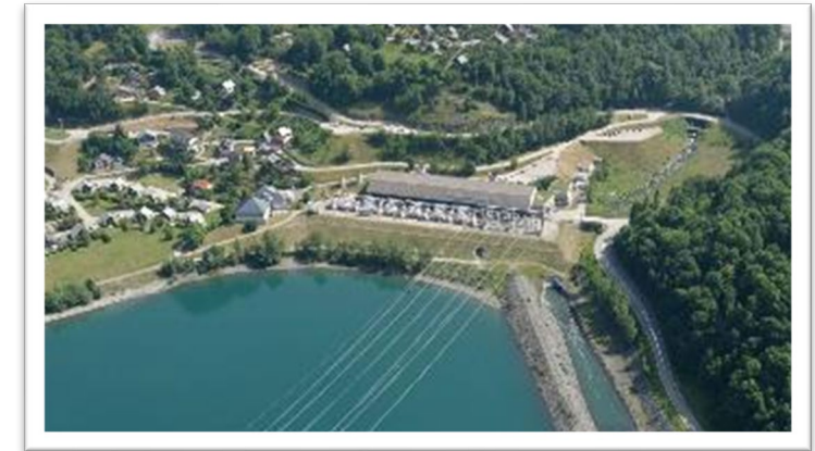
Grand Maison upper reservoir and PSH plant – 1,800 MW (France) © EDF
