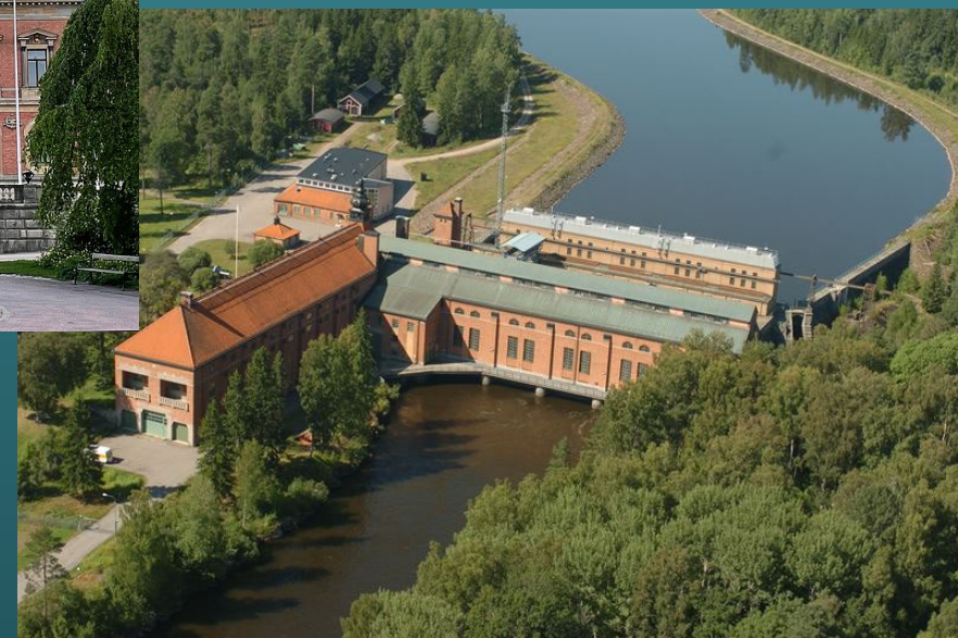
Älvkarleby Hydropower Plant
