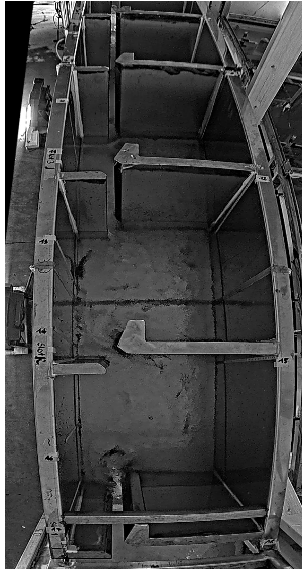
Open fishway pool 3&4
