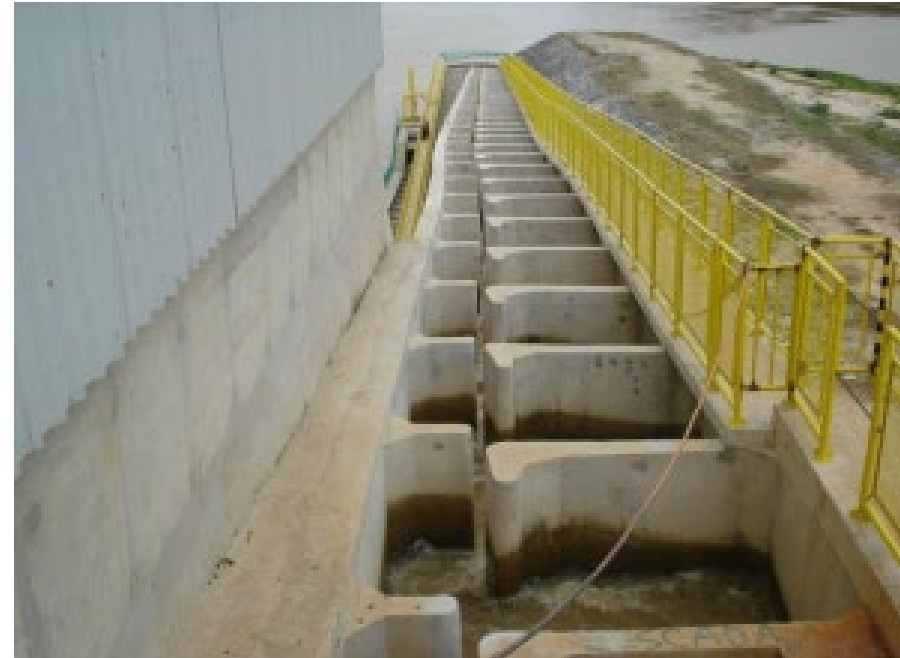
vertical slot fishway (Brazil)
