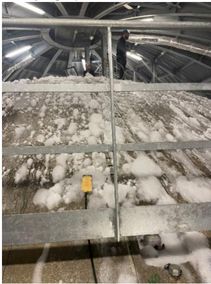
Figure 19 Applying leakage spray to the containment
