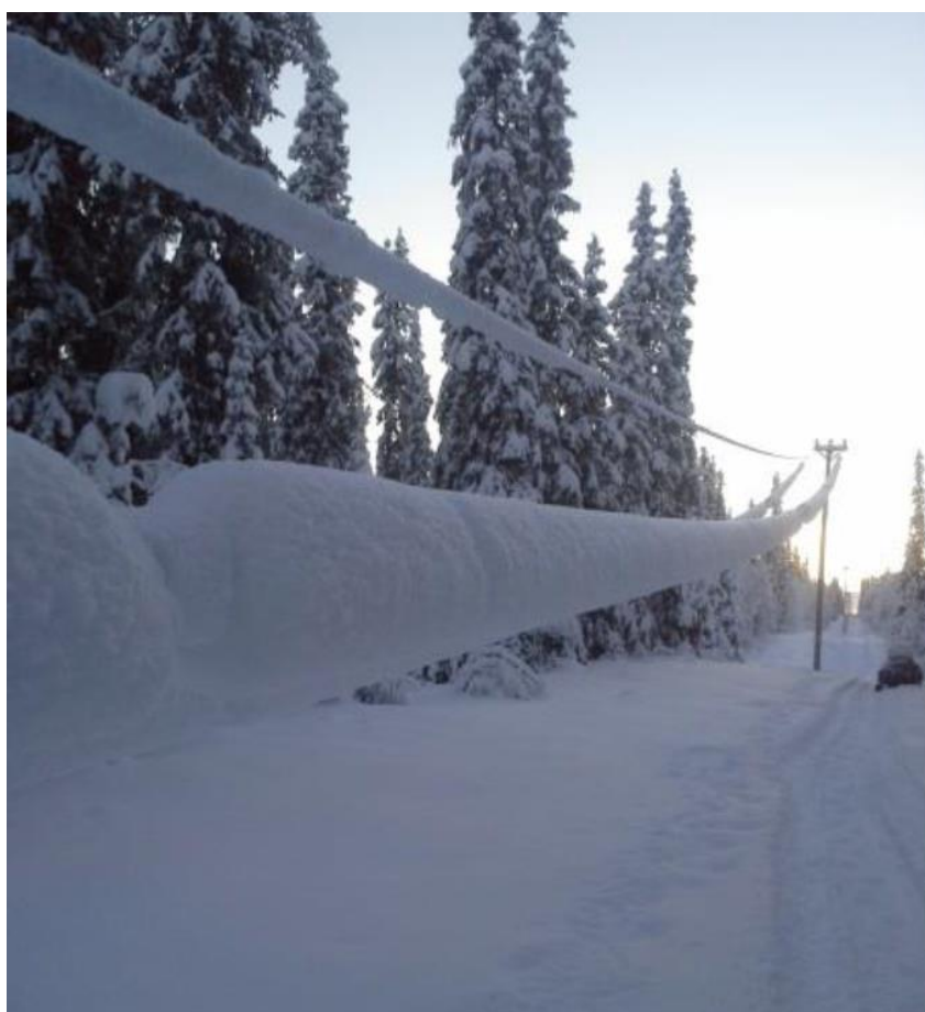
Figure 1-1. Example of ice load on a distribution line in Northern Sweden. Picture received from Vattenfall Eldistribution (included with permission).
