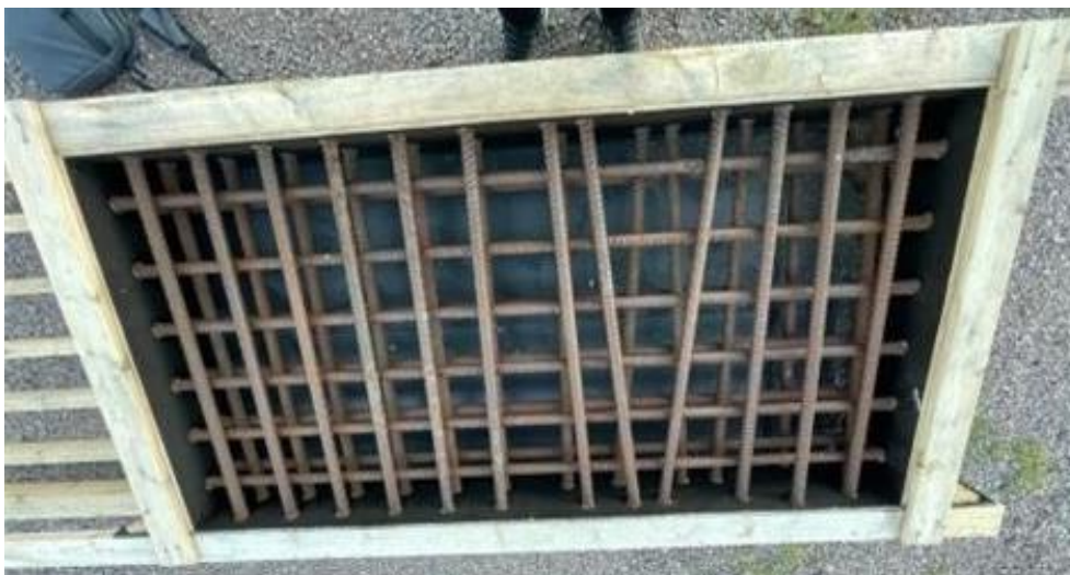
Figure 1 - Overview of the rebar layers before casting the test block.
